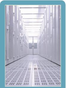
The cold aisle containment is a state-ofthe-art solution for energy efficiency and cold air distribution.
