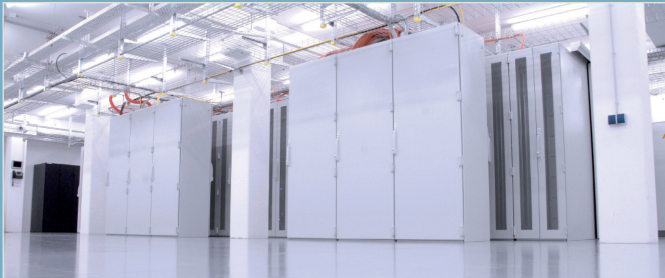
Ventilated customer racks (rear) with separate fiber and copper cable trays above. Central MMR/ODF racks (front).
